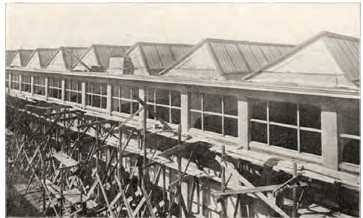
Factory Building under construction showing saw-tooth roof with large glass panes for lighting
